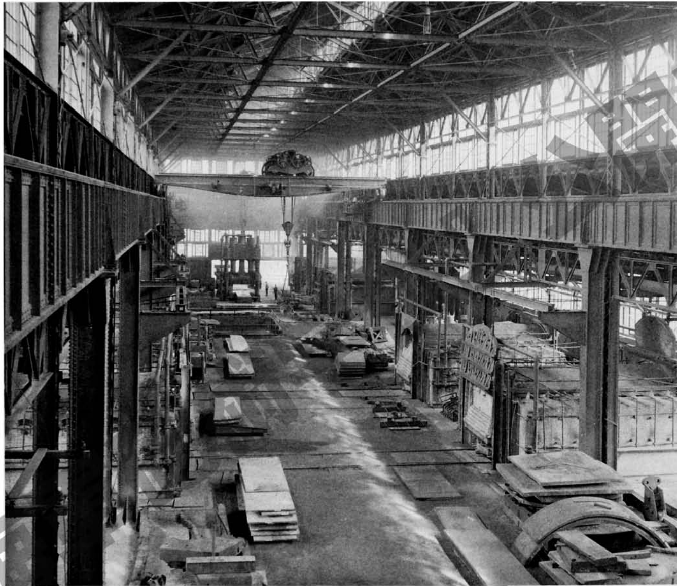
INTERIOR VIEW OF ARMOR PLATE BENDING SHOP. HOMESTEAD STEEL WORKS. ARMOR PLATE DEPARTMENT.
