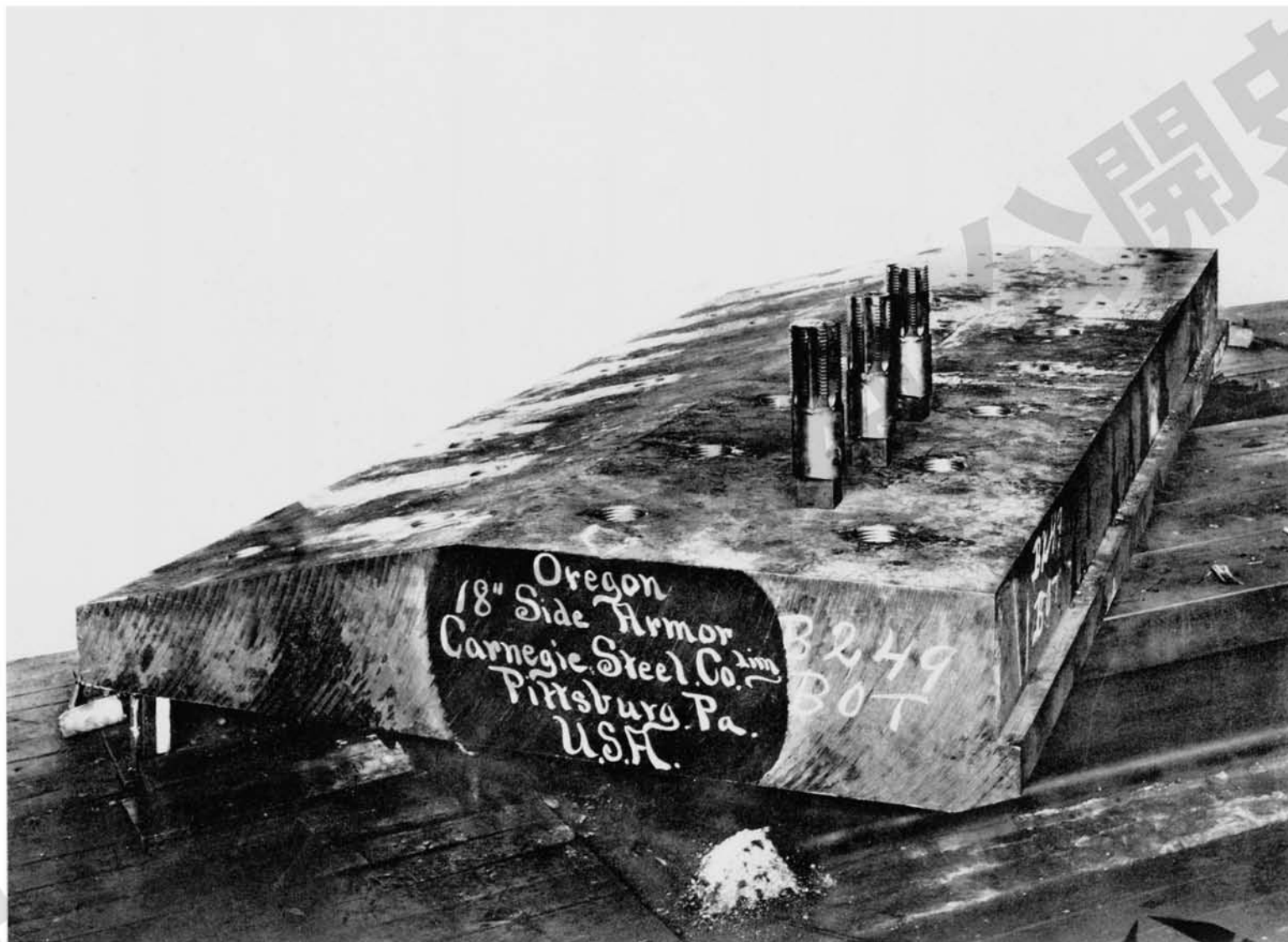
18 INCH NICKEL STEEL FACE HARDENED SIDE ARMOR PLATE FOR U. S. BATTLESHIP "OREGON."
