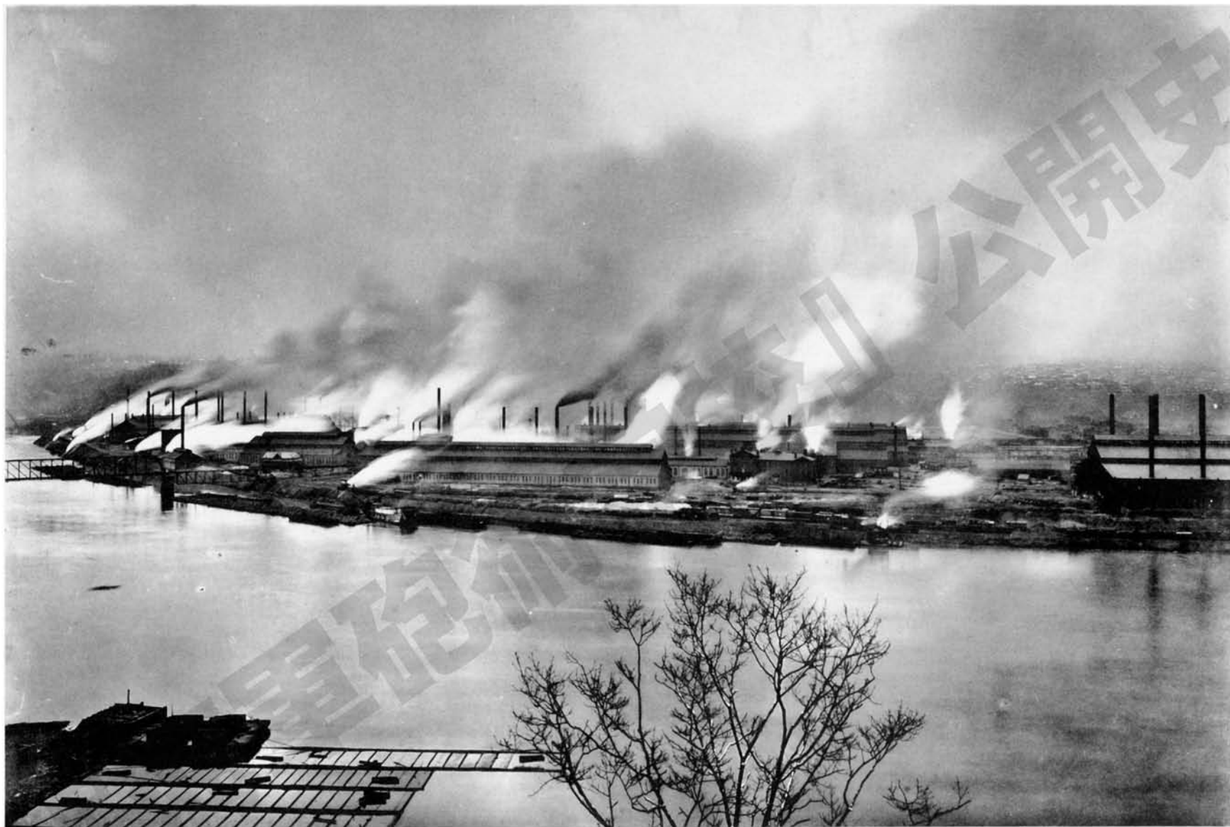
THE CARNEGIE STEEL COMPANY, LIMITED. GENERAL VIEW OF HOMESTEAD STEEL WORKS.
